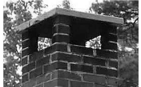
Concrete Cap Chimney Top
